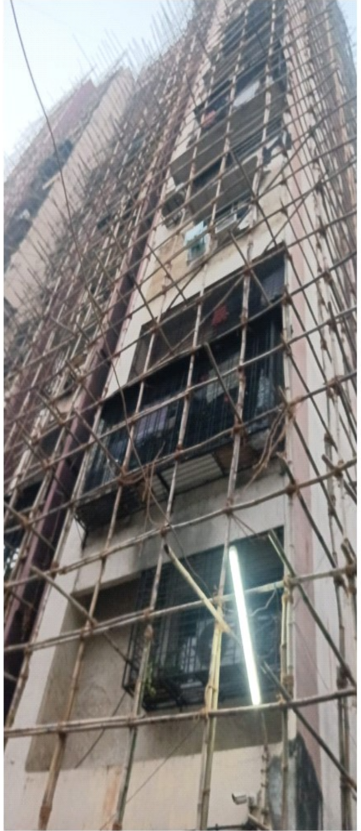
Major Structural Repairs and Restoration
