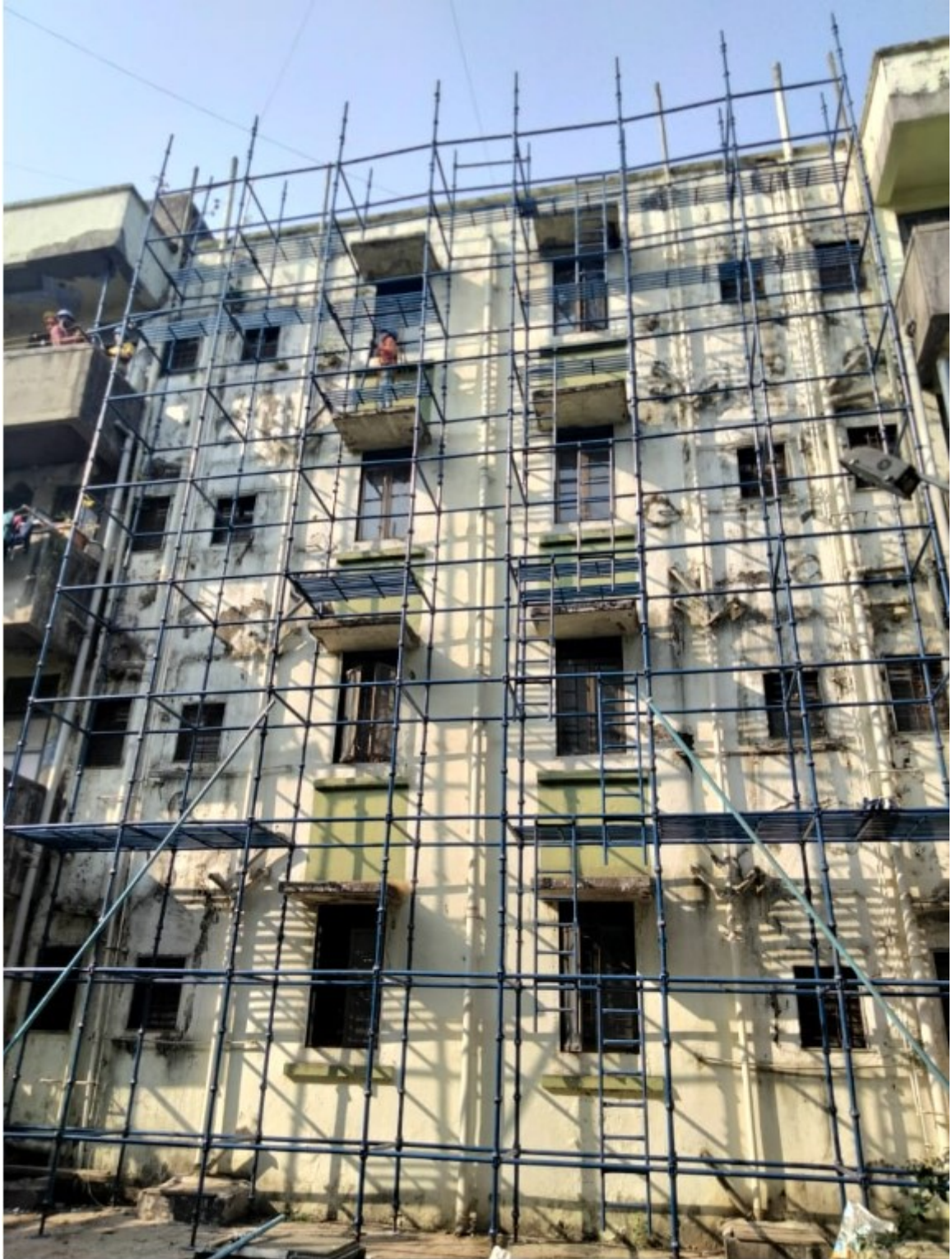
Structural Repairs and Restoration
