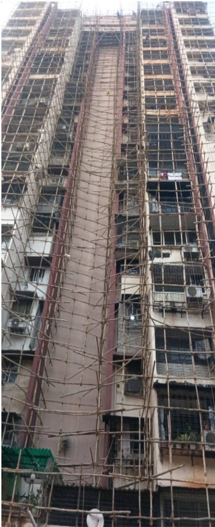
Major Structural Repairs and Restoration
